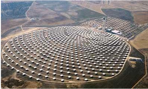
Solar thermal power station in Spain
